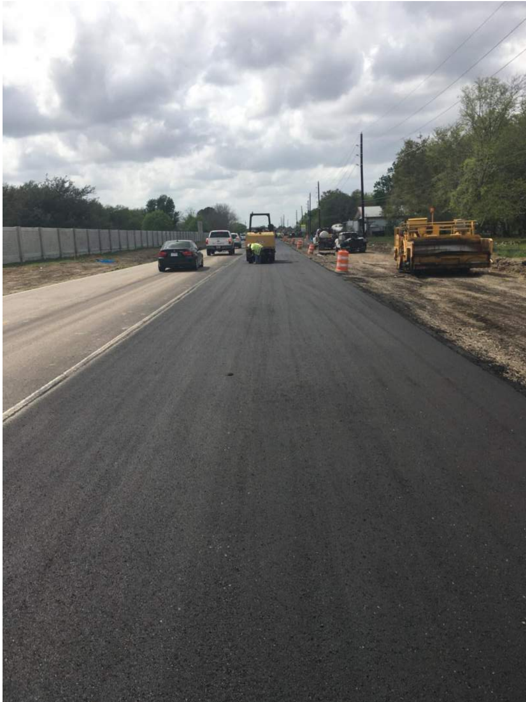
Temporary pavement finished surface facing west. 03.19.20
