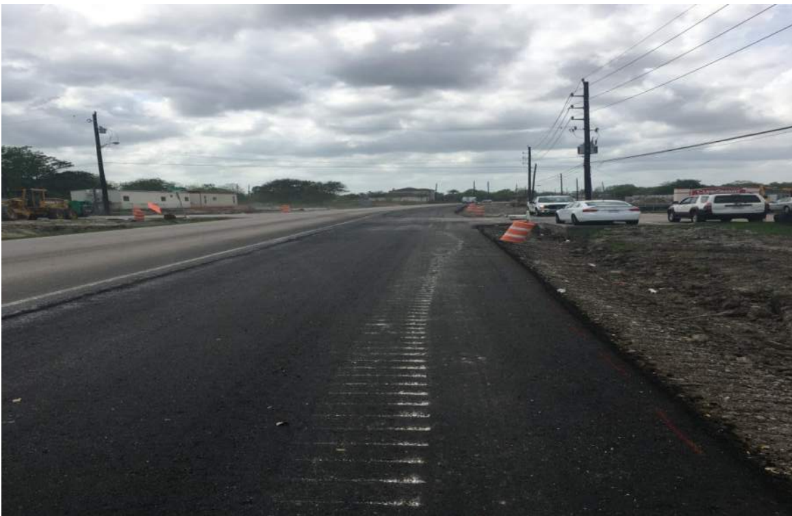
Temporary asphalt pavement. North side at Brookney. 03-19-2020
