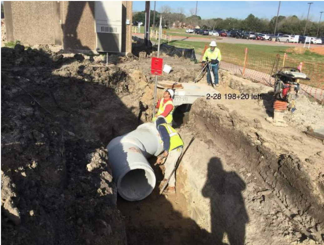
Installing storm sewer next to Dawson High behind the AT&T building. 02/28/2020
