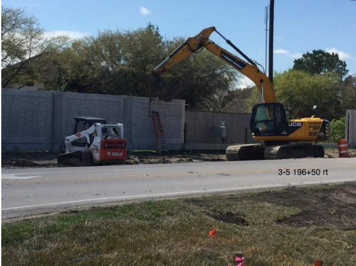
Sound wall installation at Crystal Lakes. 03/05/2020
